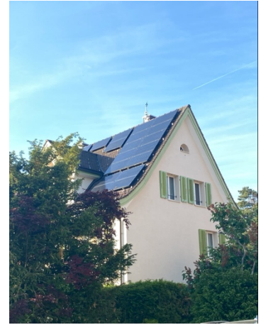
Image 2: House with solar panels in neighbourhood
