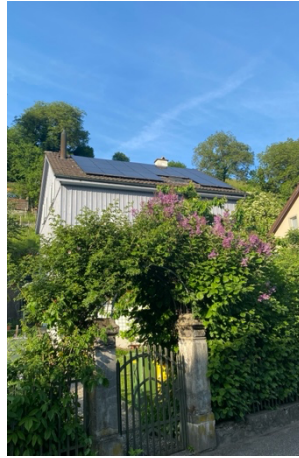
Image 2: House with solar panels in neighbourhood
